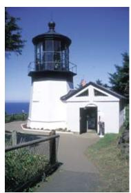
The tower light is a first order, eight-sided Fresnel lens, hand ground in 1887 by Henry LePaute in Paris. A first order lens is the largest and most powerful of the six Fresnel types. The lens was carefully loaded on to a ship that sailed around Cape Horn, then north along the Pacific Coast to Cape Meares. Workers using a hand-operated crane made from local spruce trees lifted the one-
